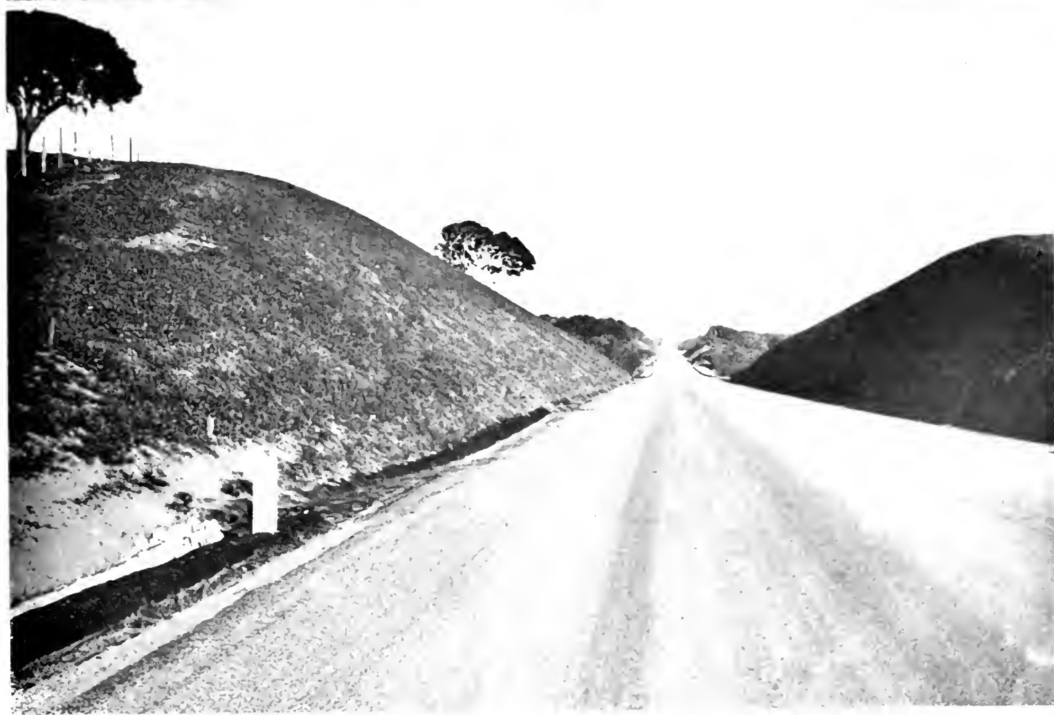
Two views of realigned and regraded sections of cut-off between U. S. 101 and coast taken before road was opened. Alignment is of high standard containing but 4 curves which have a minimum radius of 2500 feet. The 36 foot roadbed has a 22 foot plant mixed surfacing on a crusher run base and 7 foot shoulders, bituminous surface treated.
